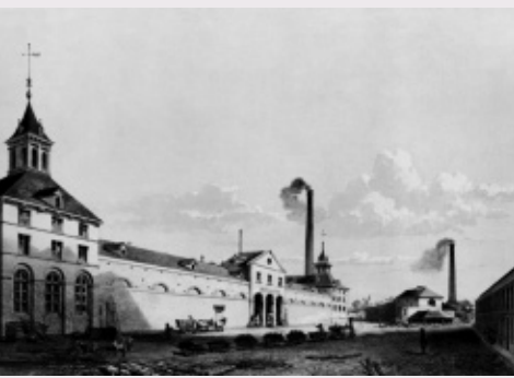
Contemporary postcard showing the industrial installations at Le Grand-Hornu
