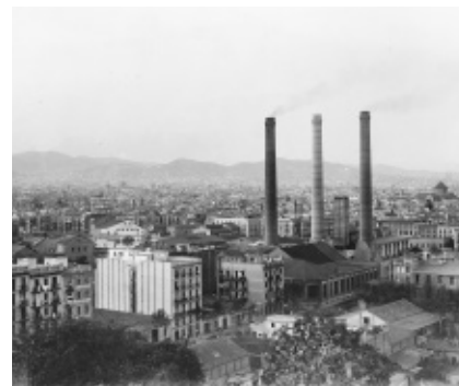
The Canadiense plant with its iconic three chimneys
