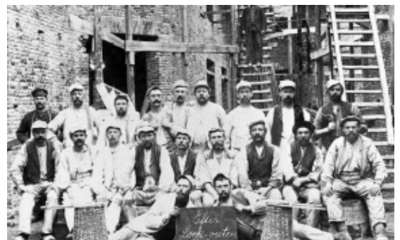
Bricklayers return to work after the conflict, which lasted almost five months.
