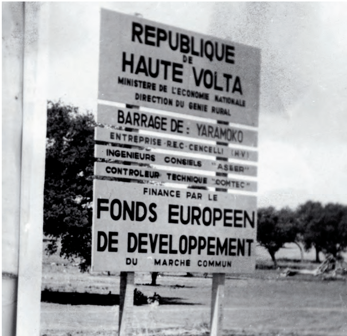
March 1965, the European Development Fund finances the construction of a dam at Yaramoko in Upper Volta (now Burkina Faso).
